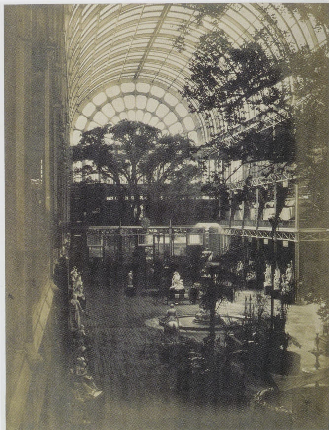
VIEW OF TRANSEPT, LOOKING SOUTH.
