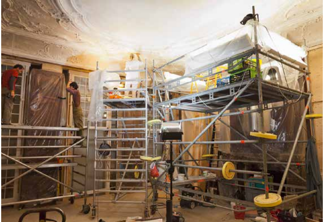
Fig. 17 Installing the new frames and making good the plaster layer as part of the installation of the room in the Rijksmuseum. Photo: Amsterdam, Rijksmuseum, HA-0029047.
