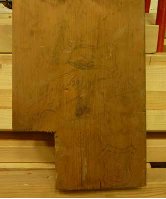
Fig. 3a Inscription on a beam on which the ceiling was suspended in the Stedelijk Museum: 'Stedelijk Museum Johan Zikking 20 September 1896 Stad Amsterdam' with the arms of Amsterdam twice.
