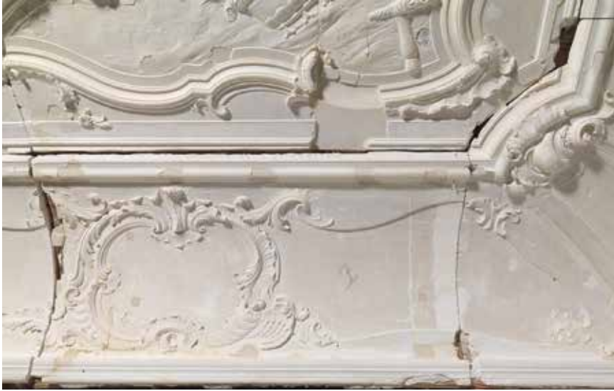
Fig. 13 Corner of the ceiling during the trial set-up in the Rijksmuseum repository. The individual ceiling elements have been consolidated, and holes or missing pieces have been filled with lime plaster. The finishing plaster layer, mouldings and ornaments were completed after the ceiling was installed. The white areas are earlier restorations with gypsum plaster.
