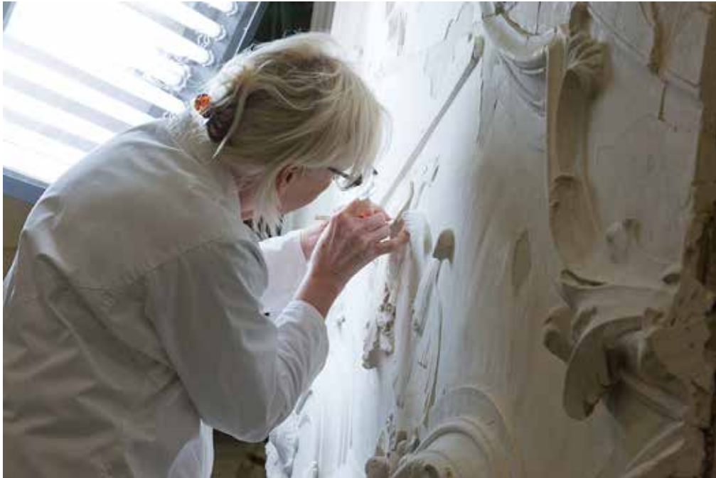
Fig. 12 Marie Huys using a scalpel to remove later coats of whitewash from the original plasterwork. Photo: Amsterdam, Rijksmuseum, HA-0022610.
