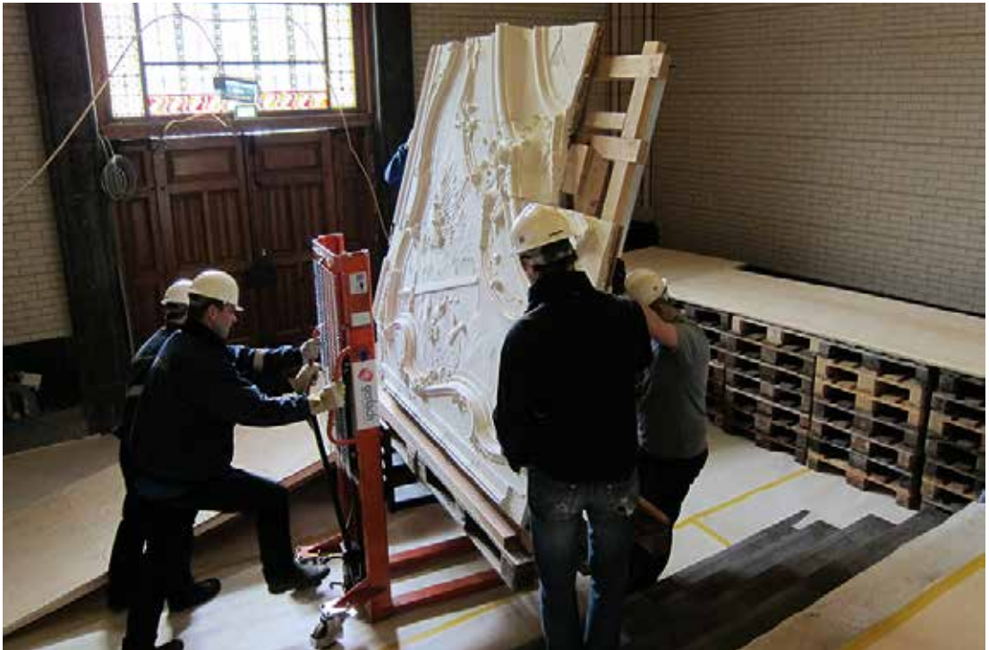
Fig. 14 Transporting the largest section of the ceiling through the Rijksmuseum's former main east entrance, 12 April 2012.
