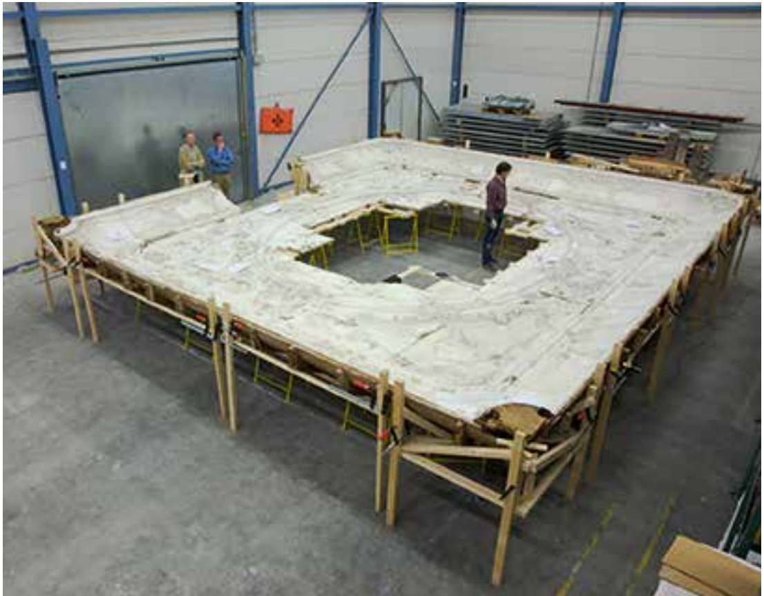
Fig. 7 After the Stedelijk Museum beams had been removed and the structure and plasterwork consolidated, the ceiling was placed on trestles to establish the correct dimensions and shape of the ceiling – and thus the floor plan for the walls.
